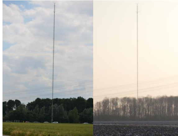
The same site during summer and winter [Project reference: MM04, Test Site Lelystad]
